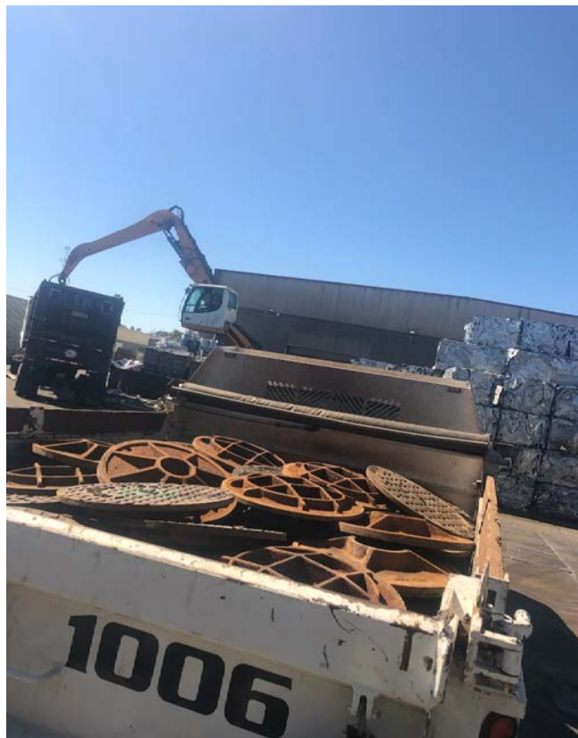
Los Altos Hills Sewer Manhole Replacement Project
