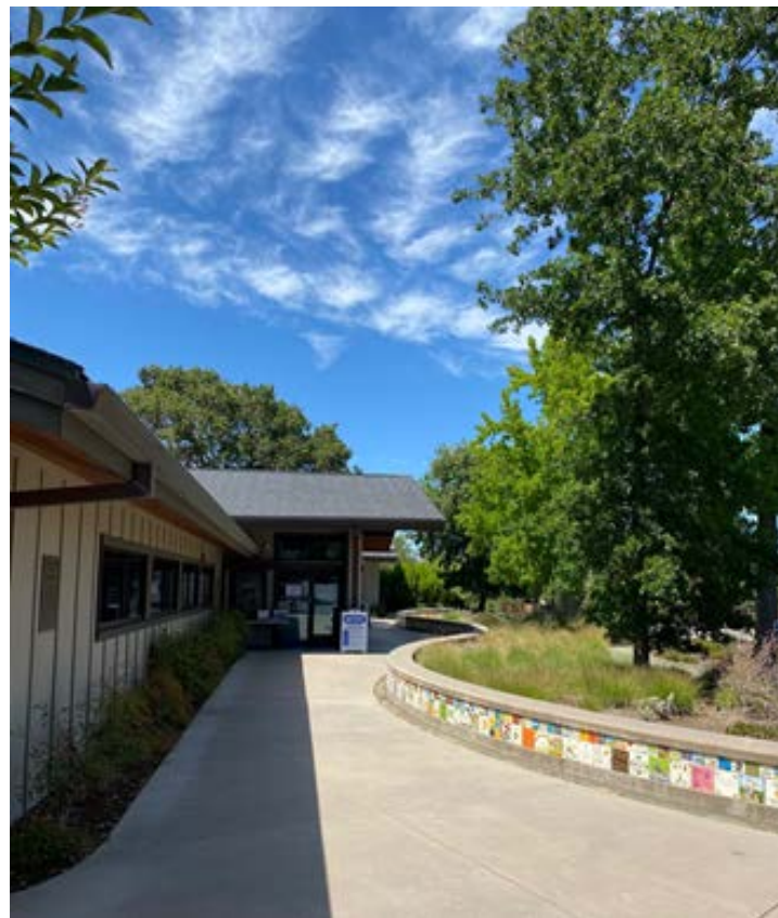
Entrance to Town Hall
