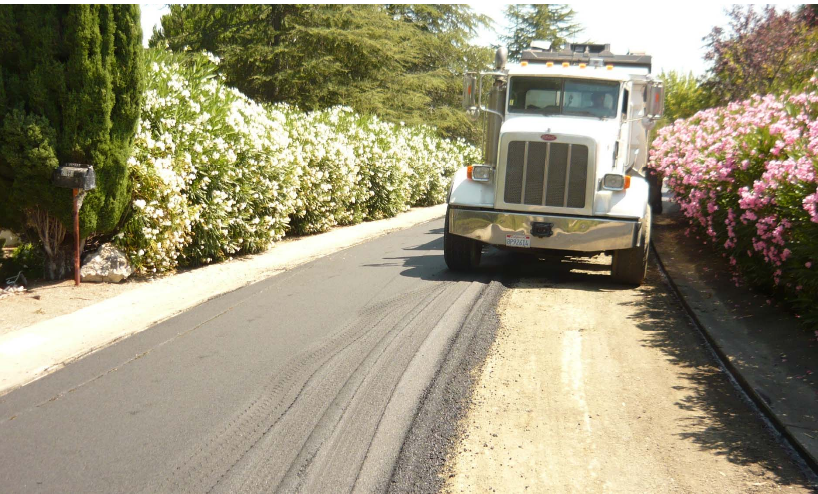
Road Rehab Project
