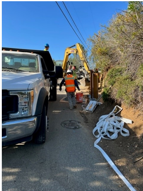
East Sunset Drive Widening Project
