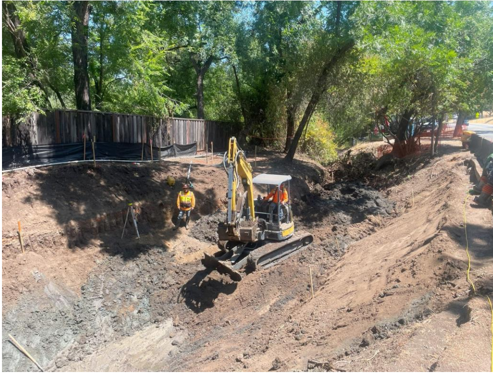
Exhibit 5: Fine Grading on Day 9 (7/11/25)
