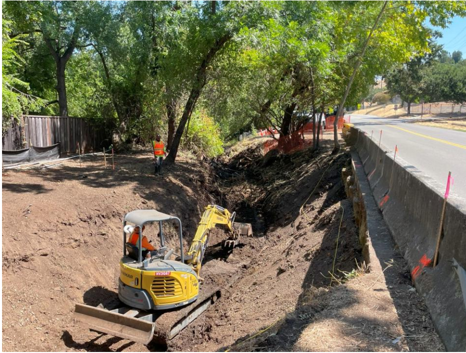
Exhibit 1: Rough Grading on Day 5 (7/7/25)
