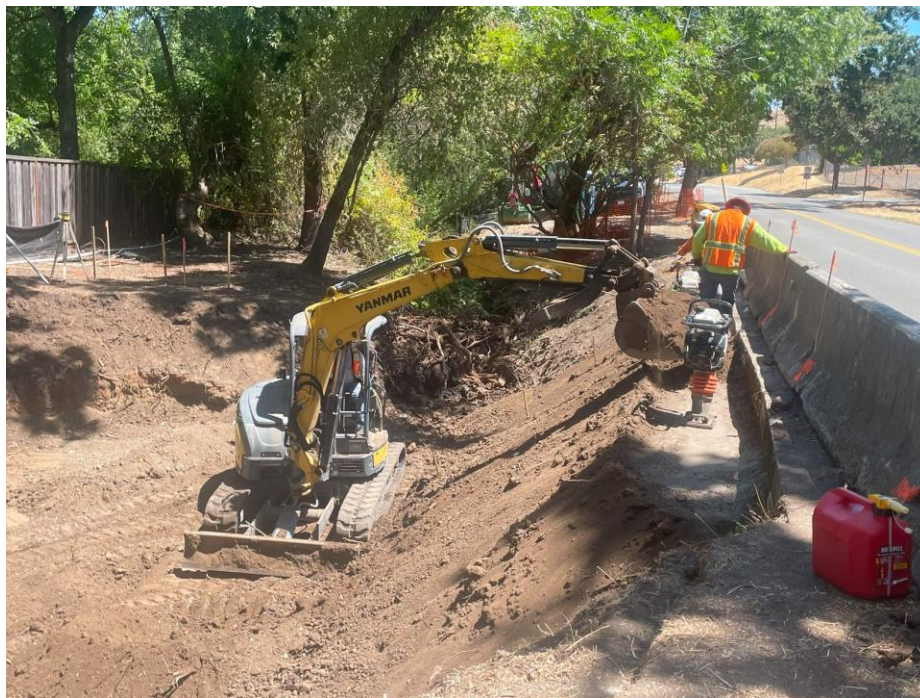
Exhibit 4: Fine Grading on Day 8 (7/10/25)
