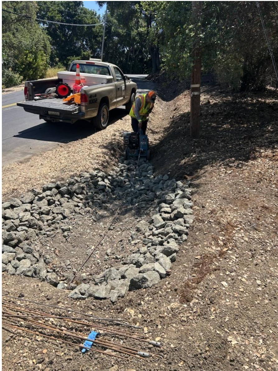
Riprap for drainage ditch on Stonebrook Drive
