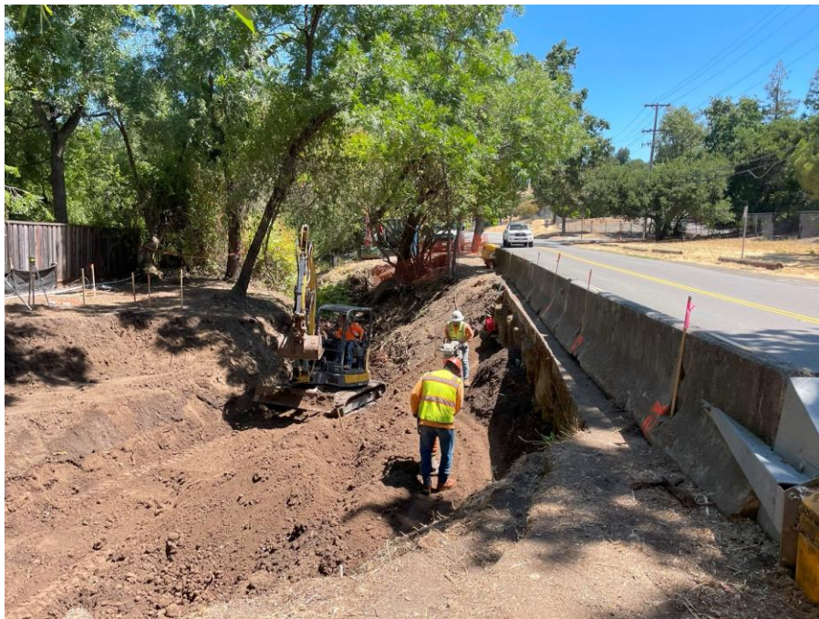
Exhibit 3: Embankment Construction on Day 7 (7/9/25)
