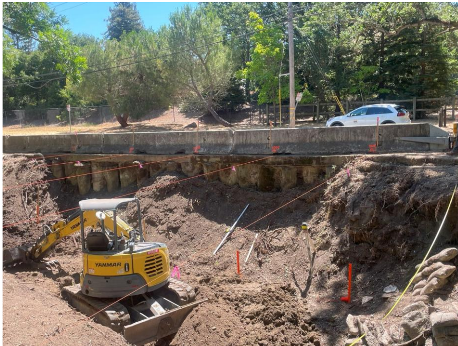
Exhibit 2: Exposed Secant Pile Wall and Survey Controls on Day 6 (7/8/25)
