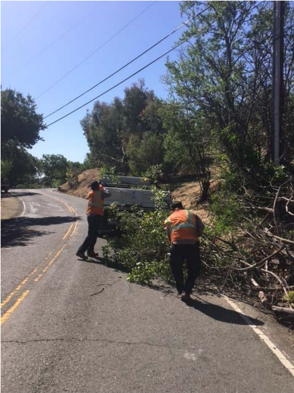
Clearing fallen tree on Elena
