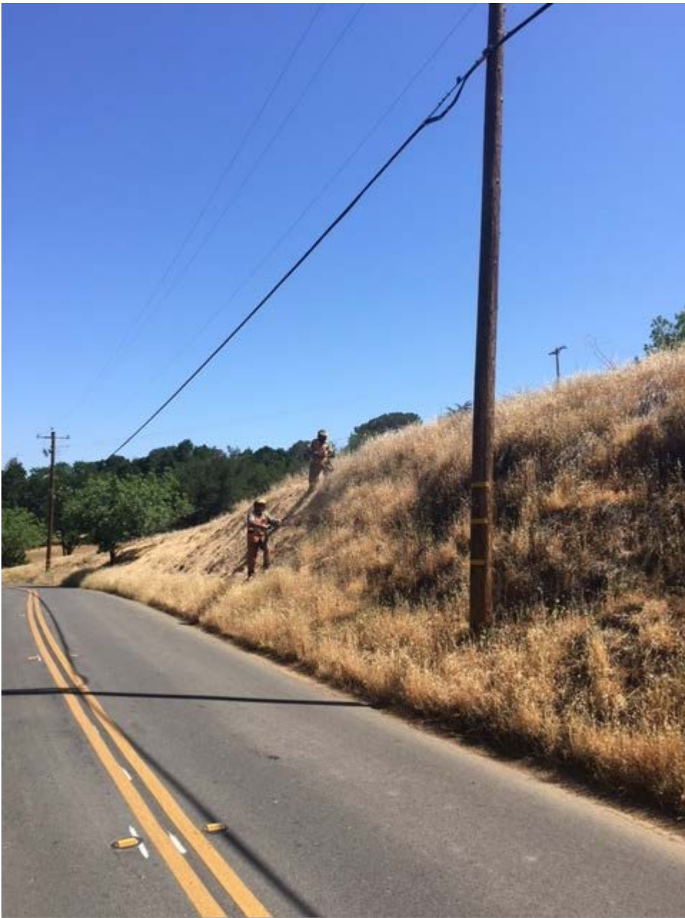
Brush clearing (before)
