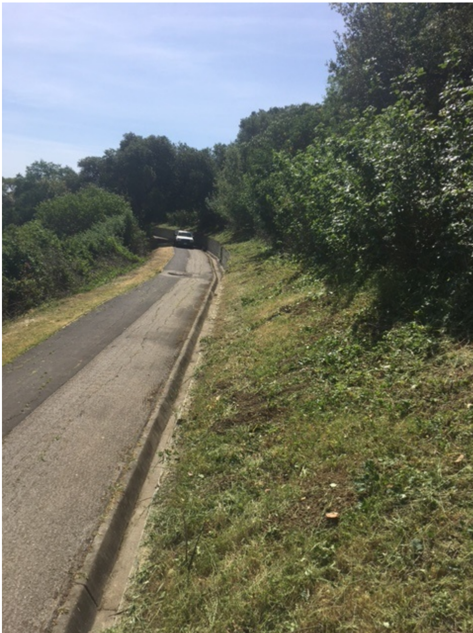
Clearing brush and tall grass for fire prevention purposes.
