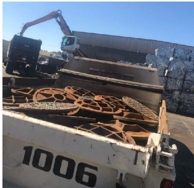
Los Altos Hills Sewer Manhole Replacement Project
